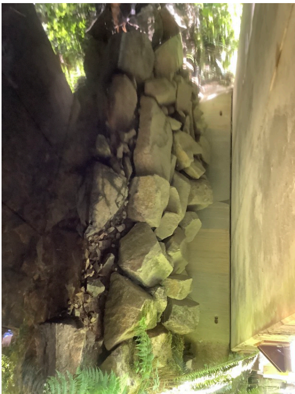
Left Bank Abutment when facing downstream
